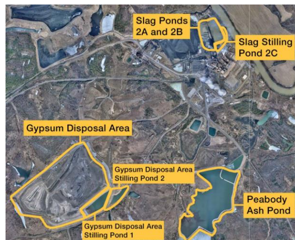
Figure 2.3 Landfills and Surface Impoundments for Coal Combustion Residuals at the TVA Paradise Fossil Fuel Plant 73
