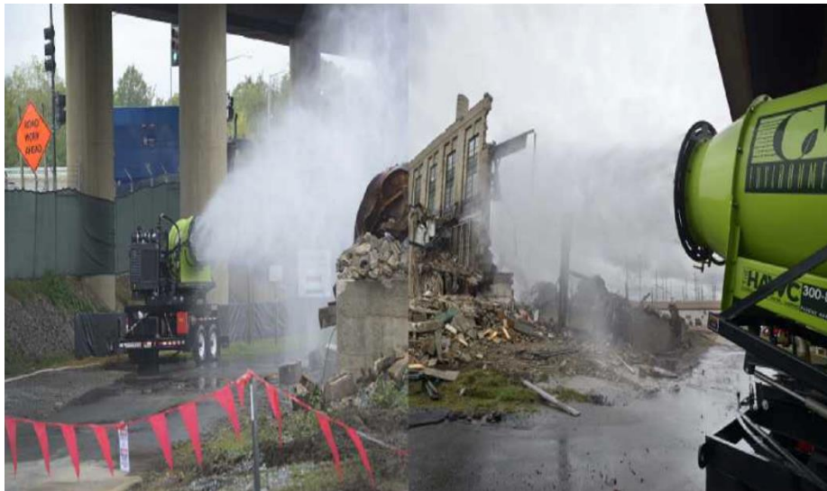
Photo 6.4. Management of Dust During Demolition 325
