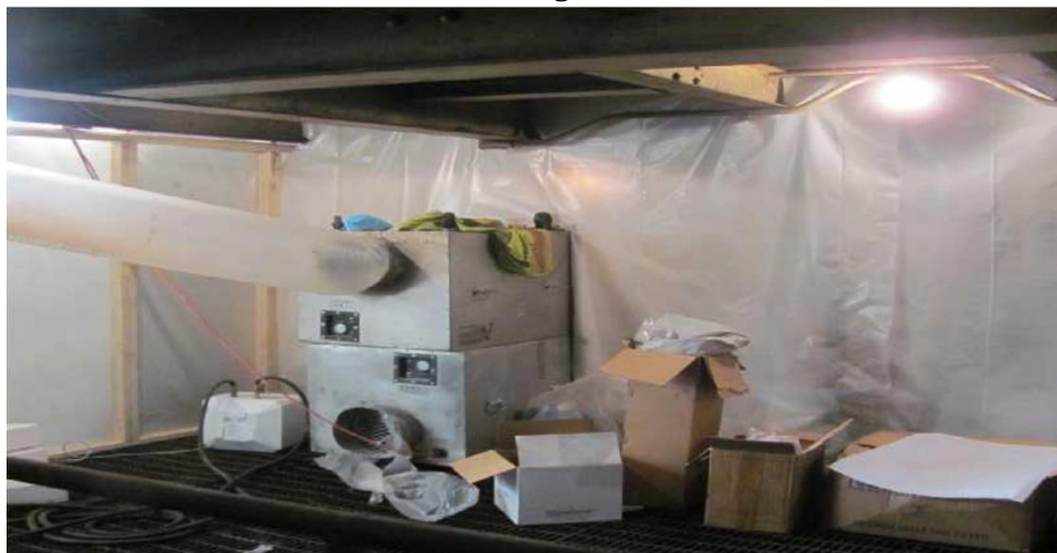
Photo 6.3. View of Asbestos Containment Area During Demolition 322
