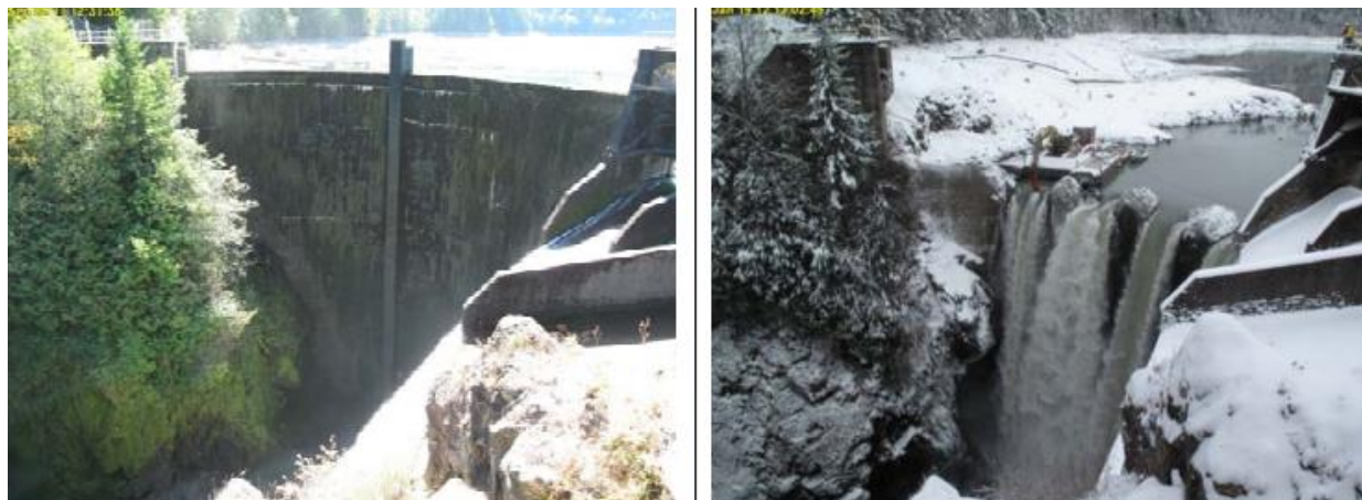
Figure 5.3. Glines Canyon Dam on the Elwha River on September 6, 2011; Removal of Glines Canyon Dam on January 19, 2012. xxv
